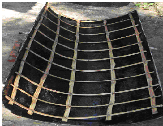
Figure 10: Progress of casting the half round bamboo reinforced precast section
