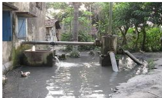
Figure 8: Head end of a deep tube well irrigation channel system
