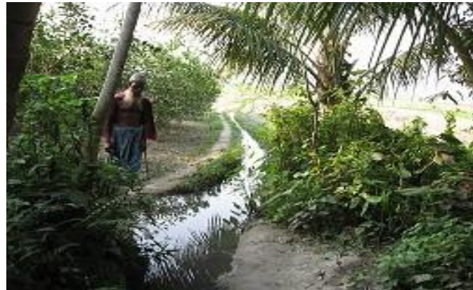
Figure 9: Drain for disposal of excess water
