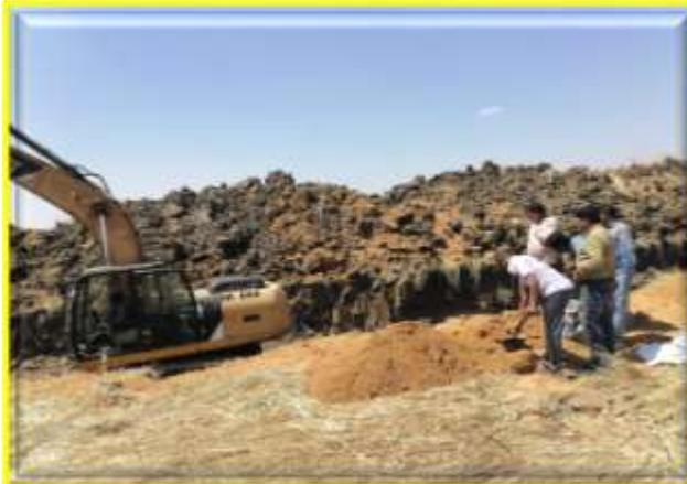
**Borrow Area Borrow Sampling Collection @ Kandamanadi Village Location @ Chainage 00 + 000 RHS Inside 2 Km Distance on the Projected Site Overburdened Removed and Stacked.**
