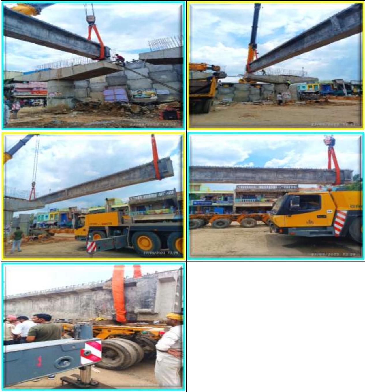
**Girder Erection Launching in Progress @ Chainage 23 + 300 Km with Construction Experts @ Viluppuram – Puducherry Section of NH – 45A (New NH – 332), Four Laning Road (Design Length Approximately 29.000 Km) in the States of Pondicherry Tamil Nadu Union Territory (UT).**
